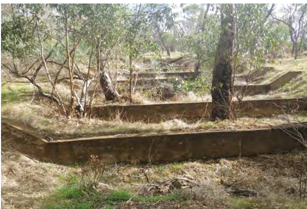
Above: Pelham waterway before and after cleanup.
